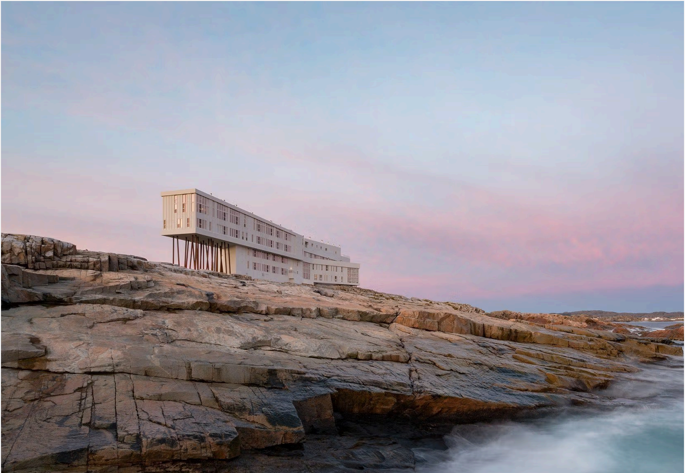
Fogo Island Inn, Newfoundland
