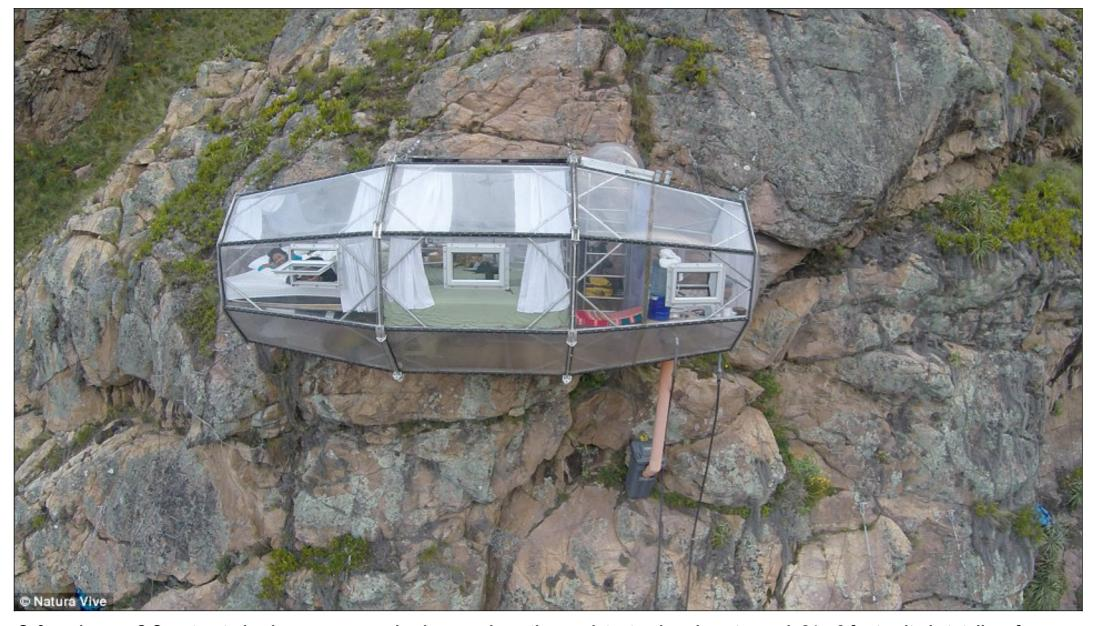
Safe as houses? Constructed using aerospace aluminum and weather resistant polycarbonate, each 24 x 8 foot suite is totally safe
